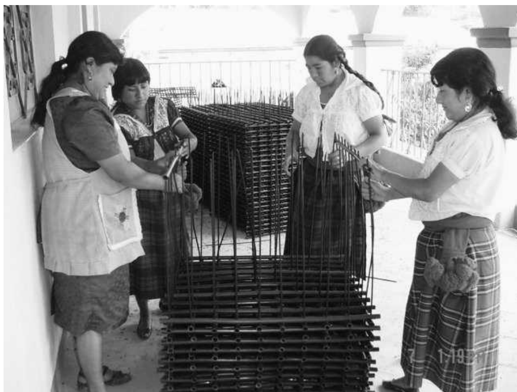
FIGURE 4 Women weaving the entrails of a community built and operated anaerobic wastewater treatment plant for recycling domestic effluents for further use for agricultural production on communal lands in a highland community in Ixtlán de Juárez, Sierra Norte, Oaxaca. (Photo courtesy of Carlos Pailles, Director, Center for Ecological Support, Huatulco, Oaxaca, Mexico)
